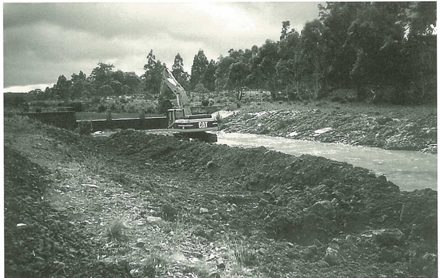
Excavator in Penstock Lagoon canal. (photo Phil Potter)
