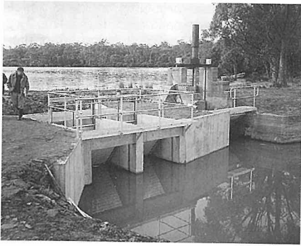
New outlet structure at Lake Sorell (photo: Tony Dell)
