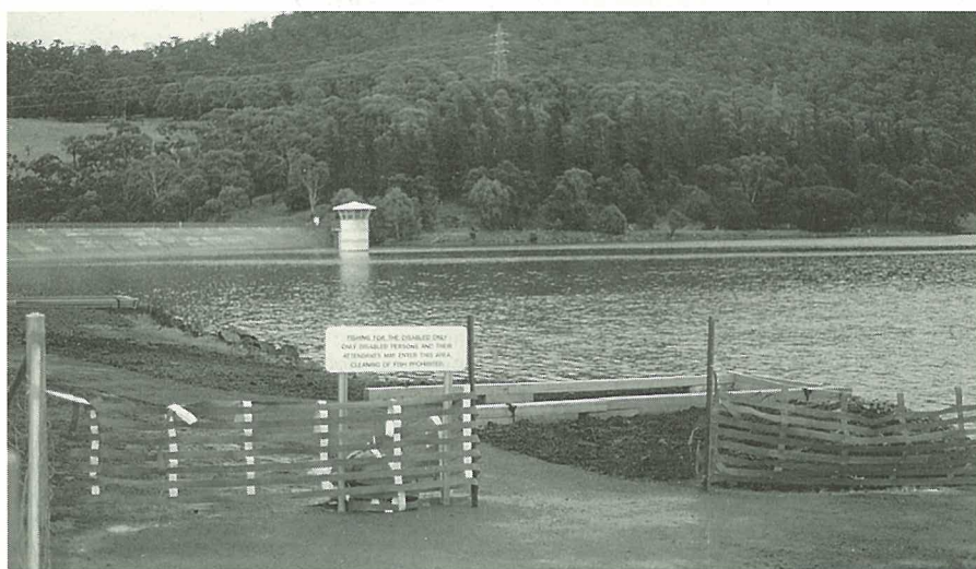
Risdon Brook dam with disabled angling area under construction
