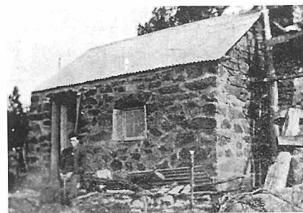
Past - during construction 1916-17 (Photo: Peter Butler)
